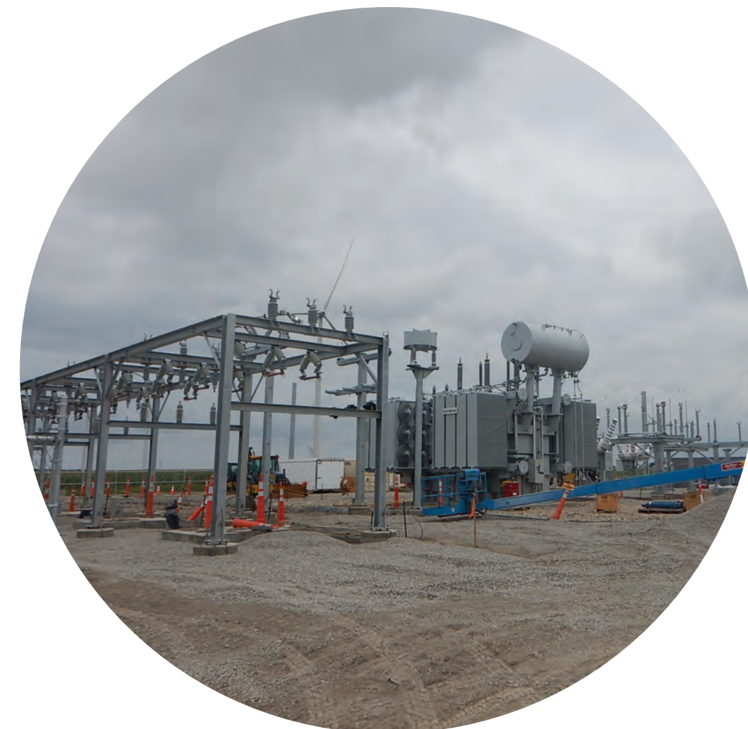
CONSTRUCTION OF ELECTRICAL COLLECTOR SYSTEM, SUBSTATION AND INTERCONNECTION POINT
