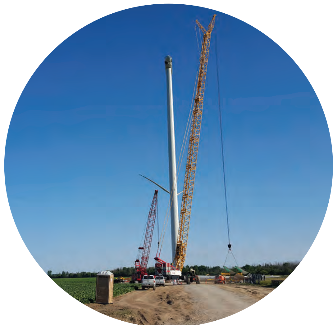
ASSEMBLY AND INSTALLATION OF WIND TURBINES
