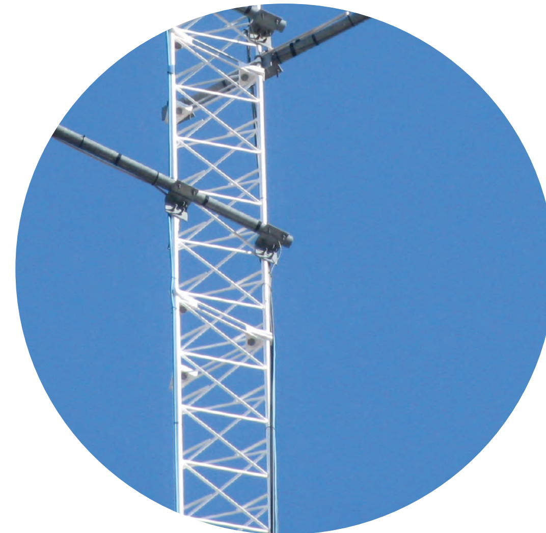
CONSTRUCTION OF COMMUNICATIONS AND METEOROLOGICAL TOWERS
