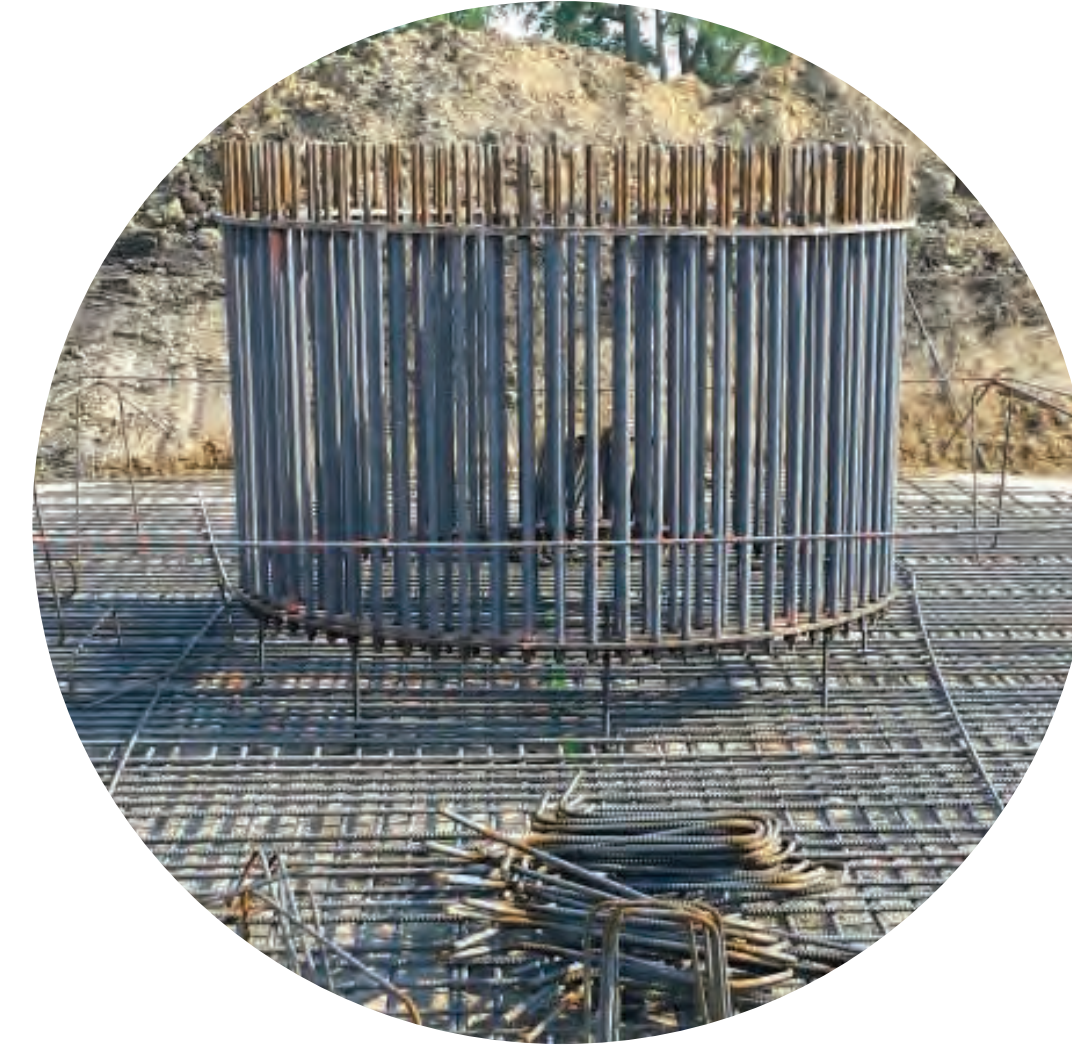
CONSTRUCTION OF WIND TURBINE FOUNDATIONS
